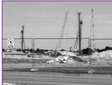
Pile drivers in action in July
