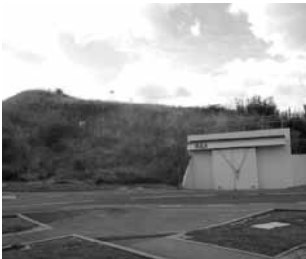
The earth mound covering the proton synchrotron of the ISIS facility. The original NIMROD synchrotron was housed in the tunnels and containments covered by the earthworks. The heavily shielded access doors to the synchrotron tunnel are particularly impressive.
