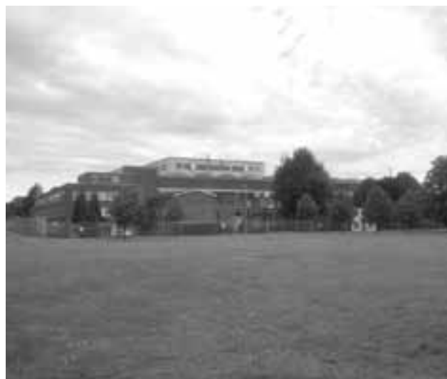
One of the original Hangar buildings (Hangar 10) from the days of the RAF Harwell airfield. The roof of the building was raised in the winter of 1947-48, with the addition of the grey box-like structure, to accommodate the BEPO (British Experimental Pile) reactor.
